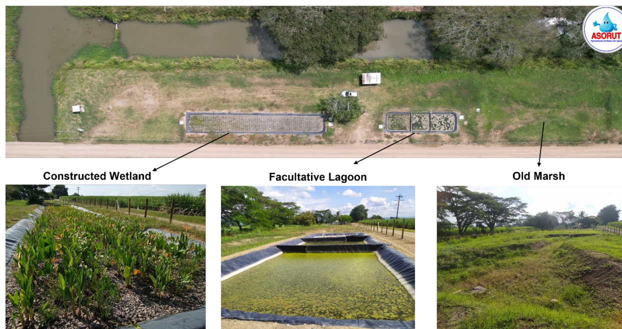
Figure 6. Nonpoint source pollution treatment pilot unit using NbS
