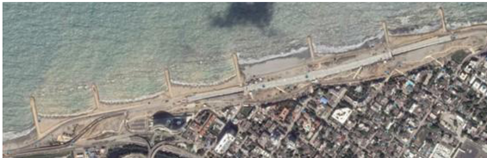
Figure 14. Satellite images of site. November 2015. Ending stage of submerge wall (33) .
