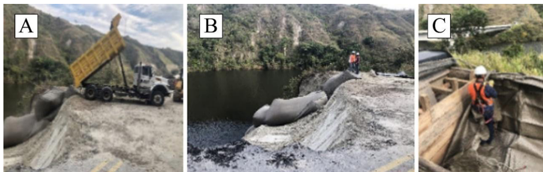
Figure 3 Bengala road recovery first stage (26)
