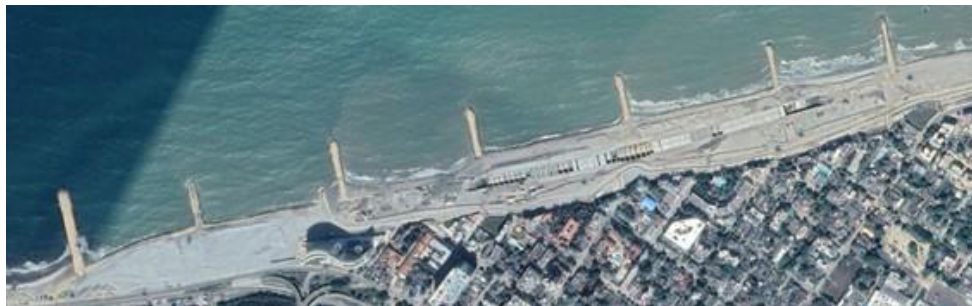
Figure 11. Satellite Images of construction site. December 2013. Final stage of seawalls construction (31)
