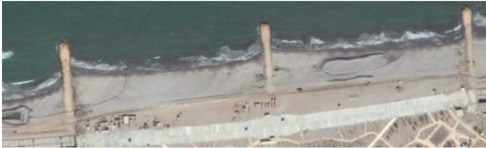
Figure 22. Satellite images. Seawalls 2 and 3. January 2016 (34)
