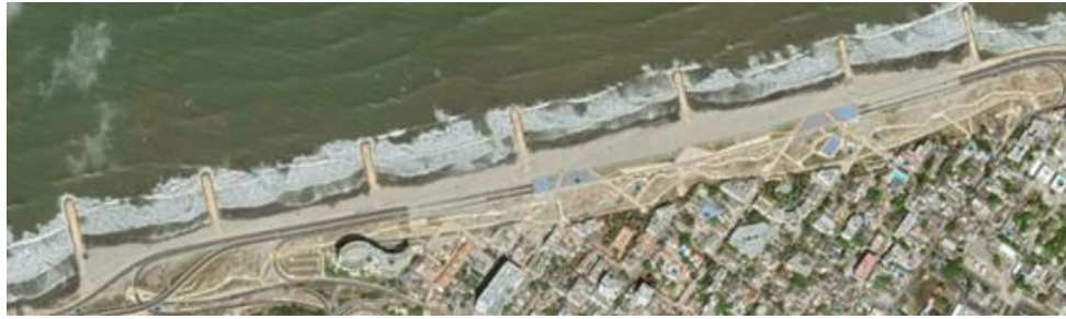
Figure 17. Satellite images of site. January 2017 (35) .
