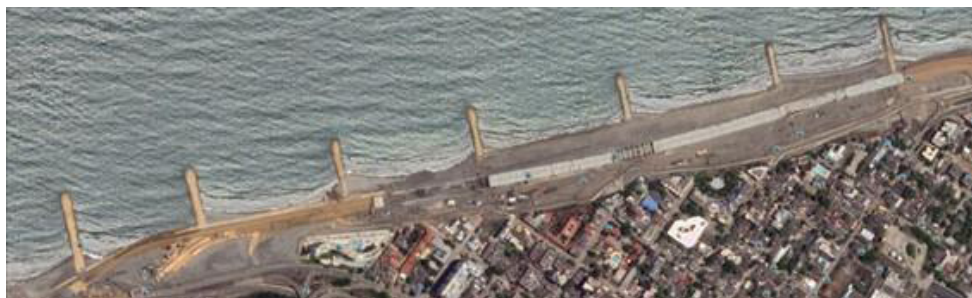
Figure 12 Satellite images of site July 2014. Added protection sand due to erosion evidence. (32)
