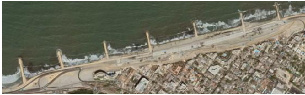
Figure 13 Satellite images of site March 2015. Beginning of submerged wall construction (33) .
