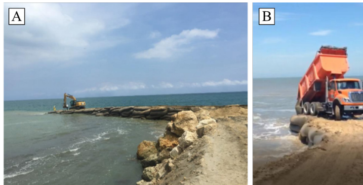
Figure 8. Submerged wall construction process (A and B)
