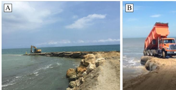
Figure 8. Submerged wall construction process (A and B)
