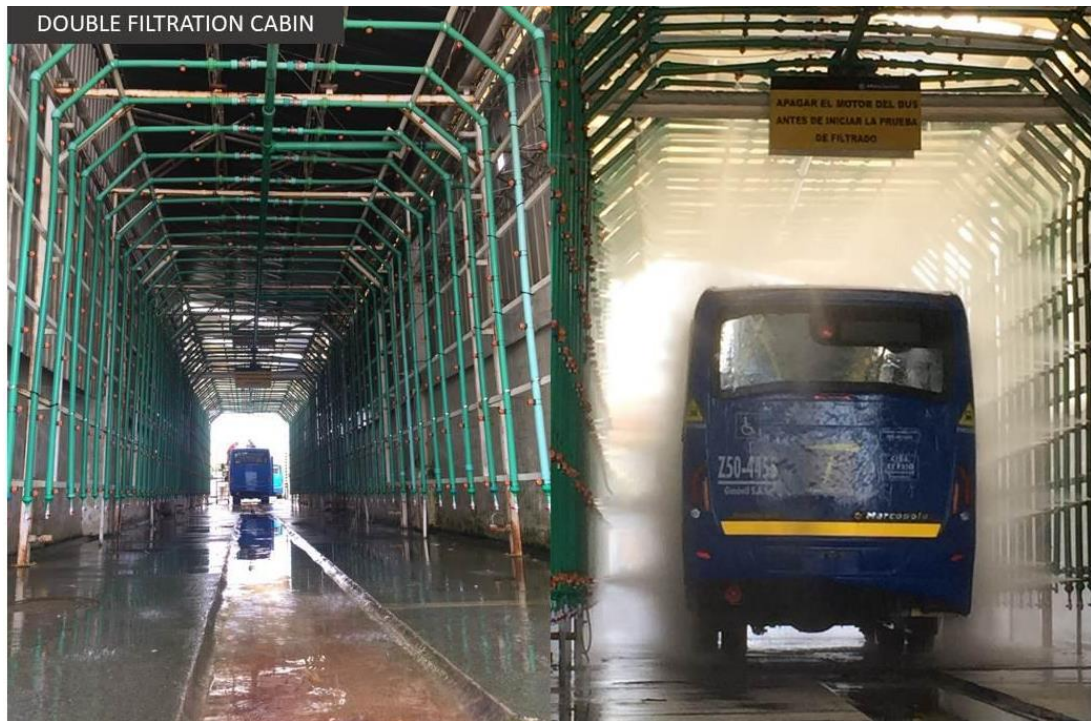
Figure 9. Leak test. Source: own elaboration
